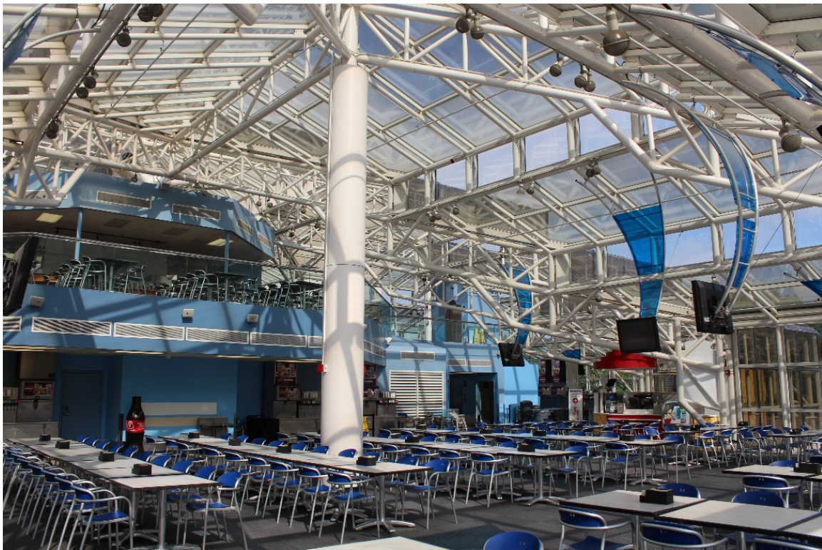
Figure 4: Restaurant addition interior, 2016 (EHT Traceries).
