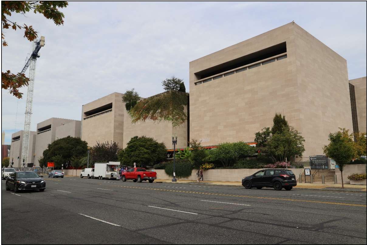
Figure 2. National Air and Space Museum, south elevation, facing northwest along Independence Avenue. New granite cladding visible at left, October 2021 (Smithsonian)
