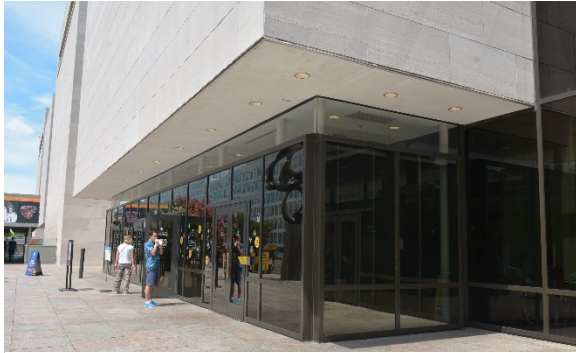
Figure 48: South entrance vestibule addition, facing northwest, 2016 (EHT Tracerics).
