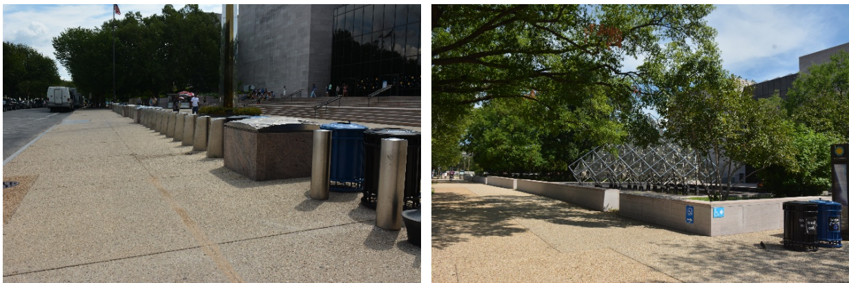
Figure 50: Perimeter security elements include bollards (above left) and the low wall along the western edge of the site (above right), 2016 (EHT Tracerics).
