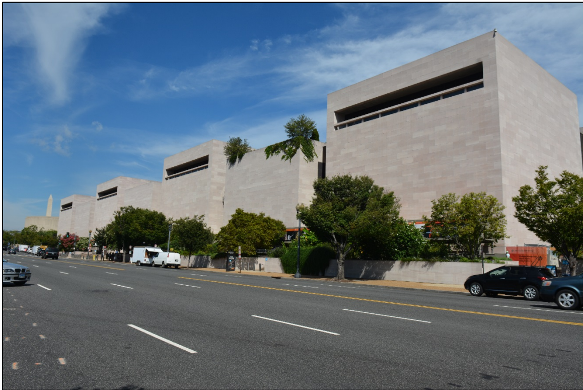
Figure 1: National Air and Space Museum, south elevation, facing northwest along Independence Avenue, 2016 (EHT Tracerics).
