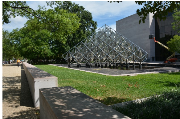
Figure 47: Delta Solar and reflecting pool, 2016 (EHT Tracerics).
