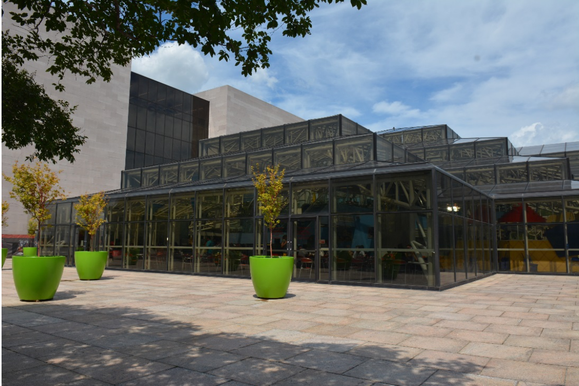
Figure 142: 1988 Restaurant addition with original building beyond, facing northwest, 2016 (EHT Traceries).
