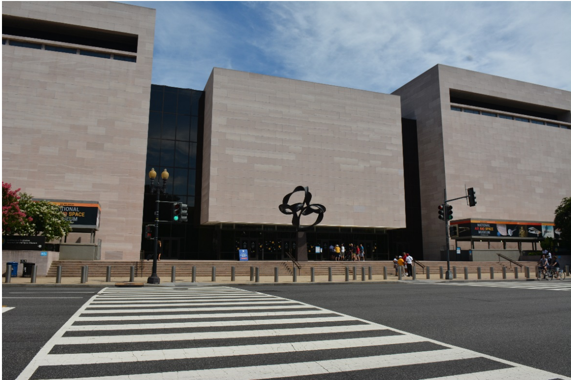
Figure 10: South elevation, cantilevered, masonry-clad block at glass bay, facing north, 2016 (EHT Traceries).
