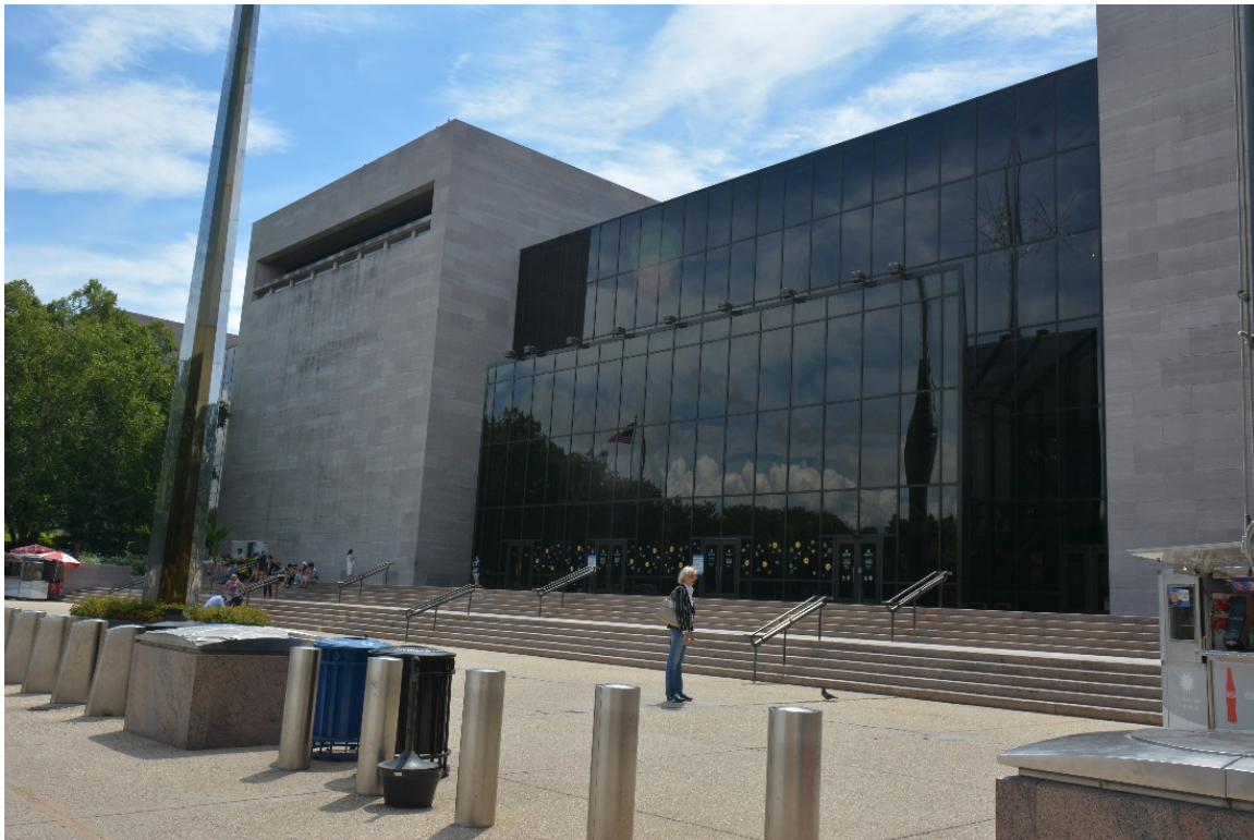
Figure 8: NASM north facade and entrance vestibule, facing southeast, 2016 (EHT Tracerics).
