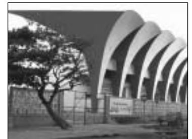
CONCRETE STADIUM CANOPY, JOSÉ MARTÍ SPORTS PARK, HAVANA, CUBA, OCTAVIO BUIGAS, 1961.
