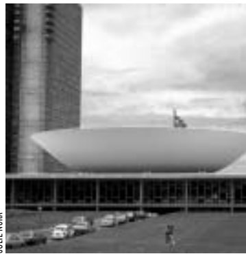
CONGRESS COMPLEX, BRASILIA (OSCAR NIEMEYER, 1958) SHOWN WITH TOWER CLADDING REPAIR UNDERWAY
