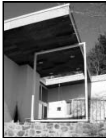
THE BUTTERFLY ROOF OF THE GAGARIN II HOUSE, BY MARCEL BREUER, FEATURES AN UNUSUAL SUPPORT.
