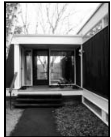
A TRANSPARENT ENTRYWAY LINKS THE TWO WINGS OF THE HUVELLE HOUSE, DESIGNED BY JOHN JOHANSEN.
