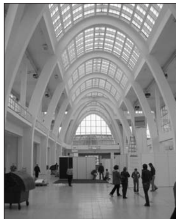
Early portion of the Trade Fair complex in Brno, Czech Republic.
