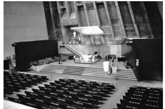
View of "floating" balcony and rear wall taken from sanctuary. (photo: Viggo B. Rambusch)
