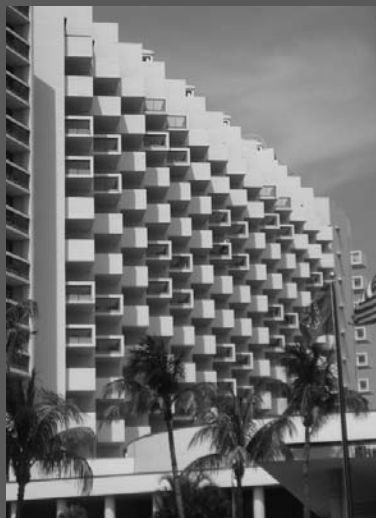
Exterior of the Sheraton Bal Harbour, Bal Harbour, FL.
