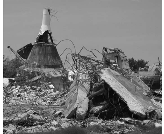
Remains of the demolition of Cabrini Church, New Orleans, LA.
