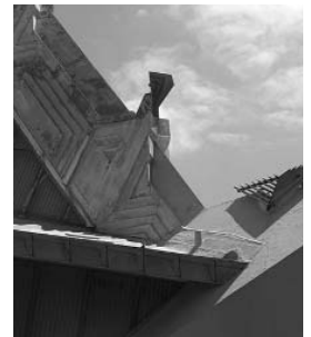
Beth Shalom Synagogue, Roof, Philadelphia, PA. (photo: Partners for Sacred Places)
