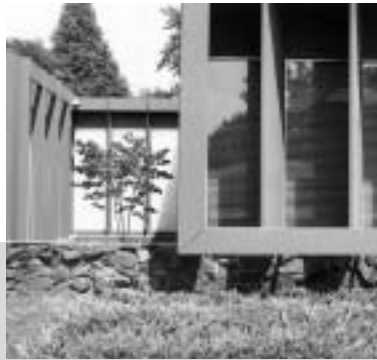
Behlen House, Columbus, NE, 1958. Detail: corrugated 16-in steel panels (photo: David Murphy, image courtesy Nebraska State Historical Society)
