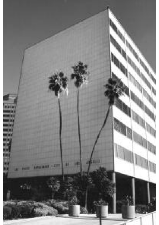
Welton Becket's Parker Building of 1959 in Los Angeles
