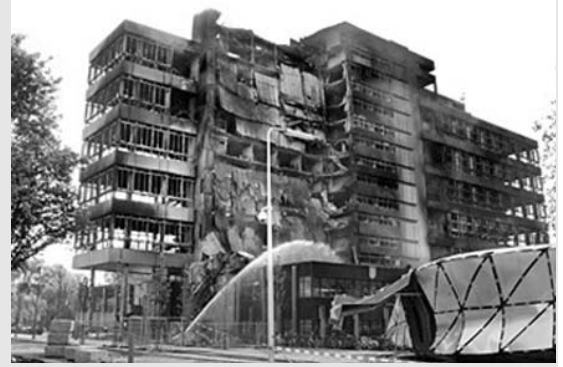
Damage to the Faculty of Architecture, Technical University, Delft. May 13, 2008 (photo: courtesy of DOCOMOMO NL)
