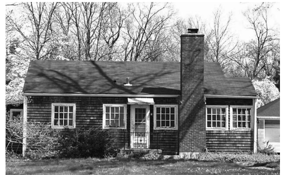
This two bedroom Gunnison Size 2-F constructed c. 1947 includes an optional Wind-O-Wing extension (to right) and working fireplace. This example is located in Lexington, Kentucky. (photo: Randy Shipp)
