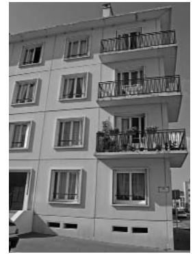
View of corner of balconies.
