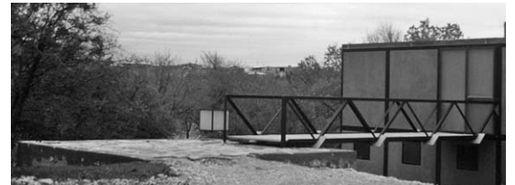
Uphill/entry side of the building. (photo: W. Mark Gunderson AIA)
