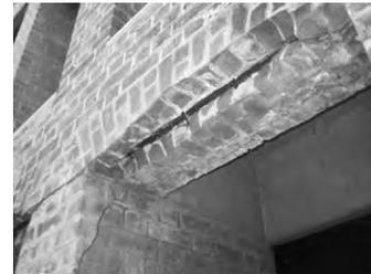
**Detail: Steel and Brick Spalling**
