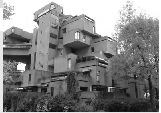
Habitat 67, Moshe Safdie (photo: Theo Prudon)
