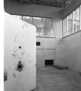
Interior, reactor room looking southeast (photo: Abby Martin)
