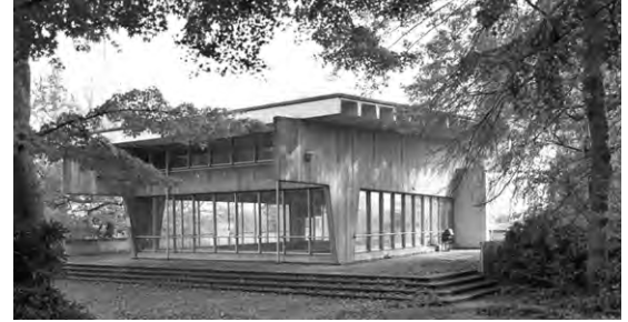
Exterior, looking east (photo: Abby Martin)
