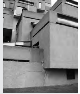
Habitat 67, Moshe Safdie (photo: Theo Prudon)
