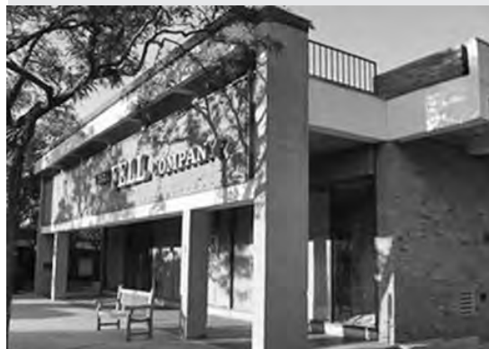
Façade. (photo: Richard Sobel)
