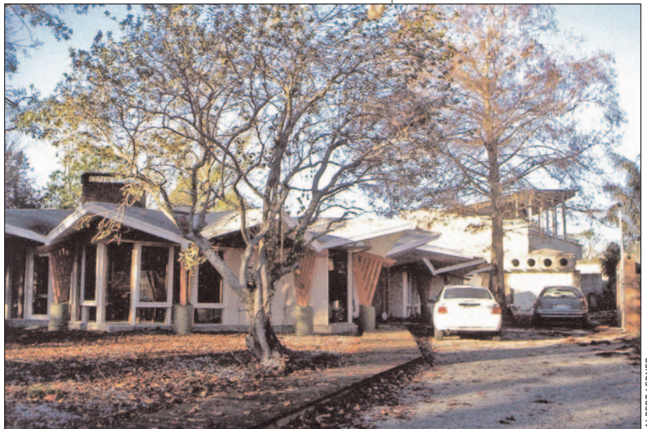
Albert Ledner's own home in New Orleans, LA. Designed in the mid-1950s, the roof form is a 12-point star supported by harp-shaped trusses resting on concrete bollards. The studio building on the right has a precast concrete first floor with a wood and plate glass second story.
